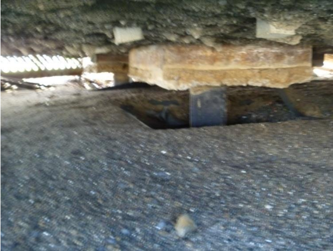
Photograph 3: Harbor Master's Office Building
