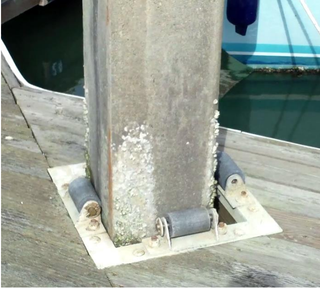
Photograph 1: Typical Pile Guide -Good Condition (Dock1)
