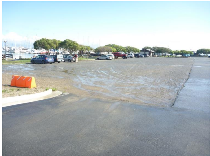
Photograph 12: Gravel Parking Lot
