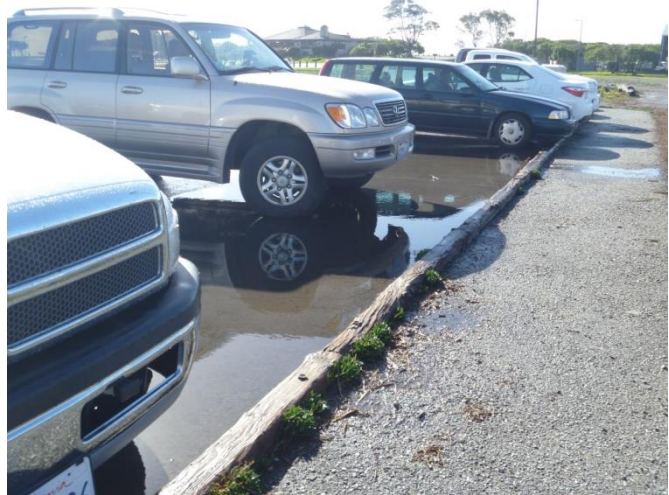
Photograph 11: Paved Parking Lot
